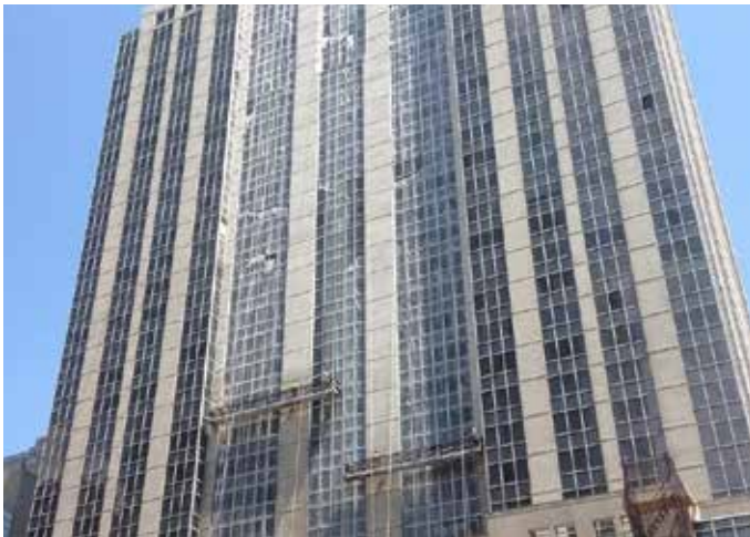
Helmsley Medical Tower NY - precast, brick, glass OneRestore high-rise
