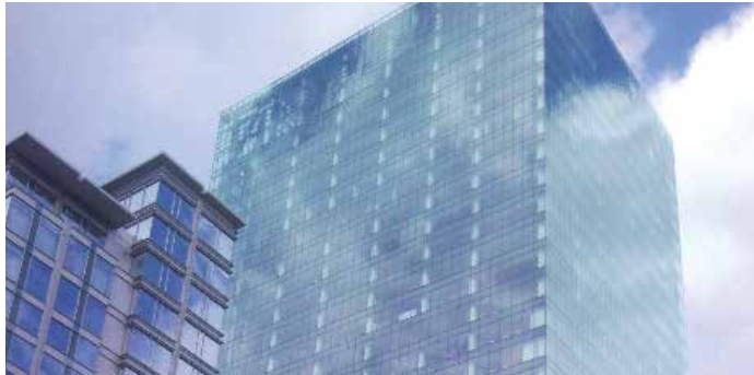
One Bank of America Center - concrete, glass, OneRestore
