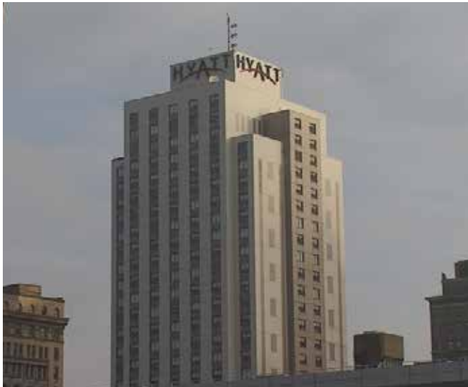
Hyatt Hotel NY - aluminum panels & precast - OneRestore high-rise
