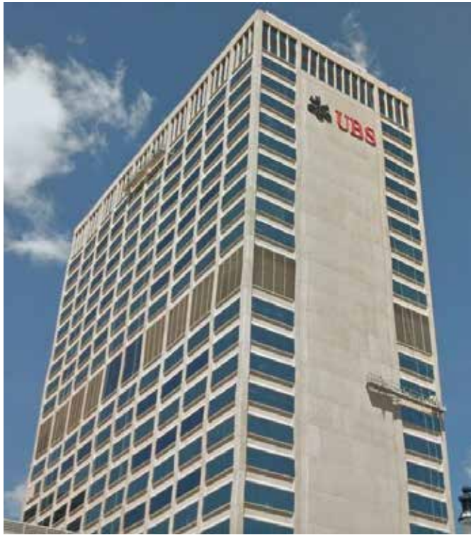
UBS Building Nashville TN precast,glass OneRestore high-rise
