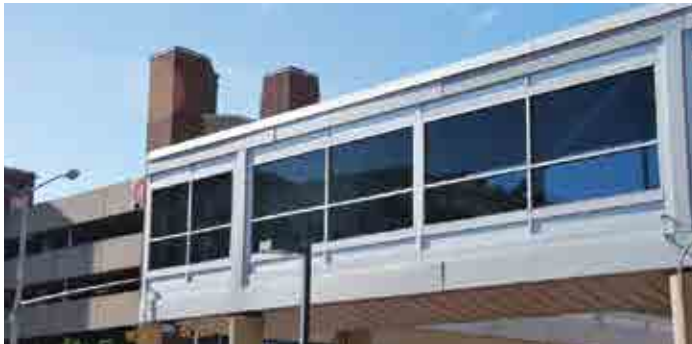
Huntsville Hospital AL, elevated walkway
