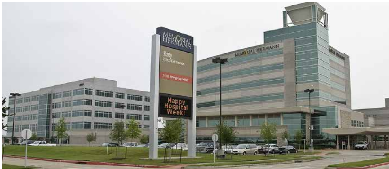
Memorial Hermann Hospital TX - painted paneling system - Cleansol BC
