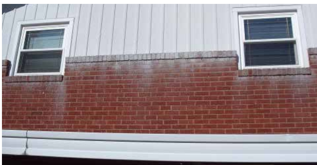
Paint wash removal from masonry.
