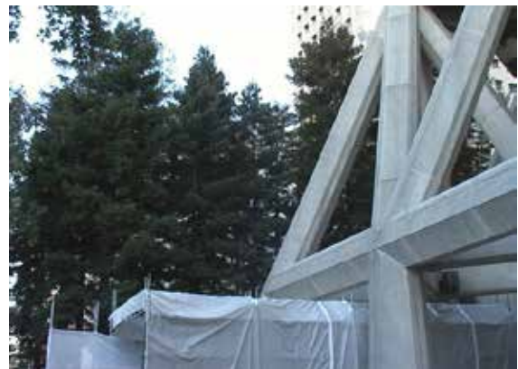
The surrounding redwood trees were far too large to cover, so this system enabled the cleaning to proceed without harming the trees.
