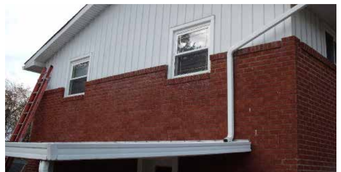
Paint wash removal from masonry.
