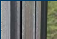
Before cleaning bronze anodized aluminum window frames
