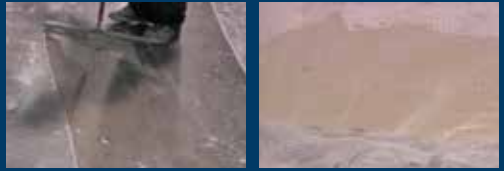
AcrylicStrip removing cured compound
