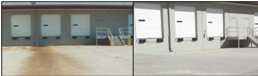
Before and after shots of a parking lot that was stained by rust and cleaned with an application of EaCo Chem's GSR followed by NMD 80.
