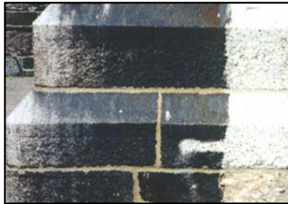
Pollution stains were cleaned from the right side of this granite with GSR.
