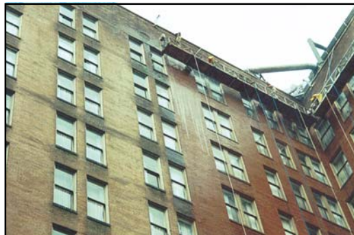
St. Joseph brick being cleaned with GSR on the Fairmont Hotel.
