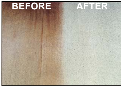
Before and after shot of rust that was cleaned with GSR.
