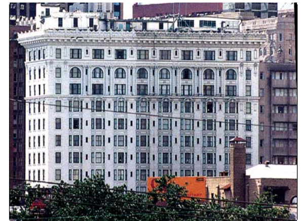
The Fairmont Hotel in New Orleans, LA was cleaned with GSR. This included the hotel's terra cotta facade.
