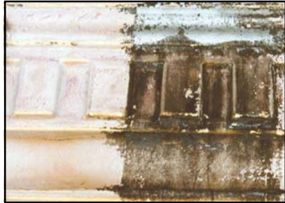
The left side of this Terra Cotta was cleaned with GSR.
